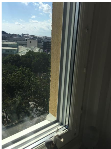
Figur 3. 2+1 isolerglasfönster.
